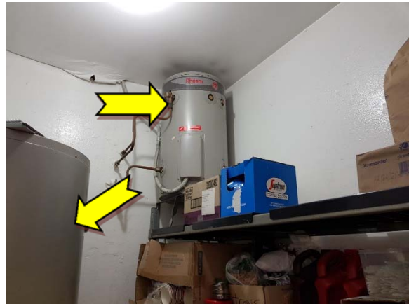
Photo 16. Interior, kitchen/kiosk, hot water heaters – suspected SMF internal insulation.
