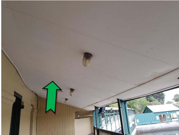
Photo 1. Exterior, level one, above kiosk, awning – non asbestos-containing fibre cement sheeting.
