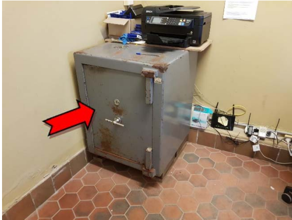
Photo 13. Interior, office, safe – suspected asbestos-containing internal insulation.
