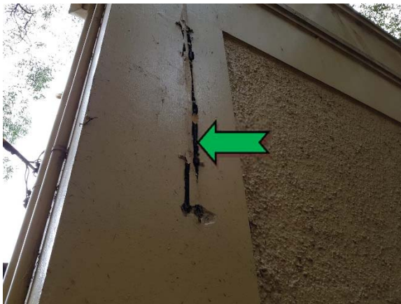
Photo 3. Exterior, north elevation, wall – non asbestos-containing bituminous material.
