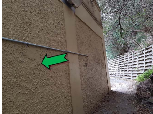
Photo 2. Exterior, north elevation, wall – non asbestos-containing textured coating.
