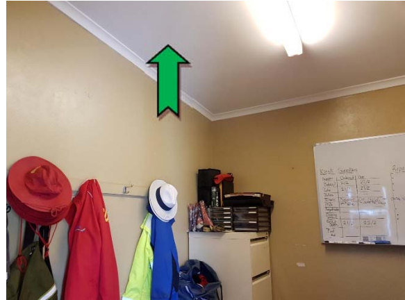
Photo 14. Interior, office/first aid room, ceiling – non asbestos-containing fibre cement sheeting.
